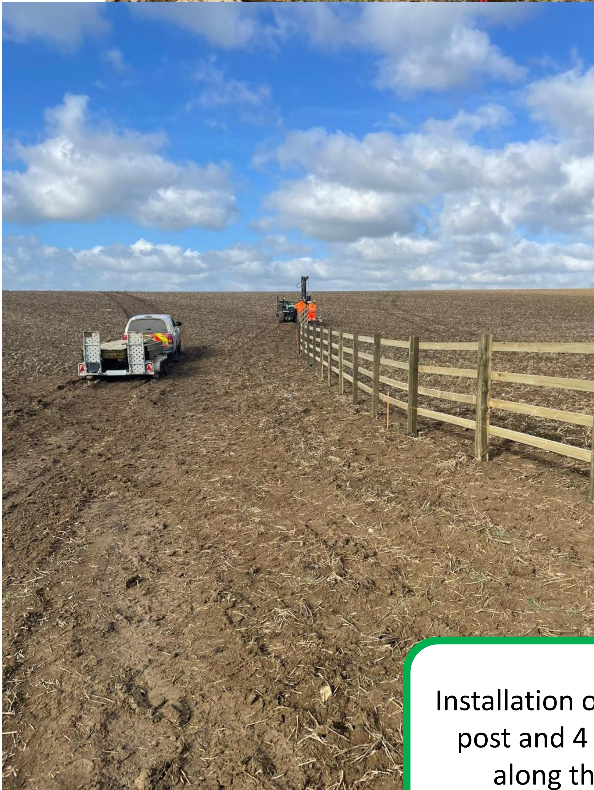
Installation of temporary fencing along the interface at the main junctions throughout the scheme route.
