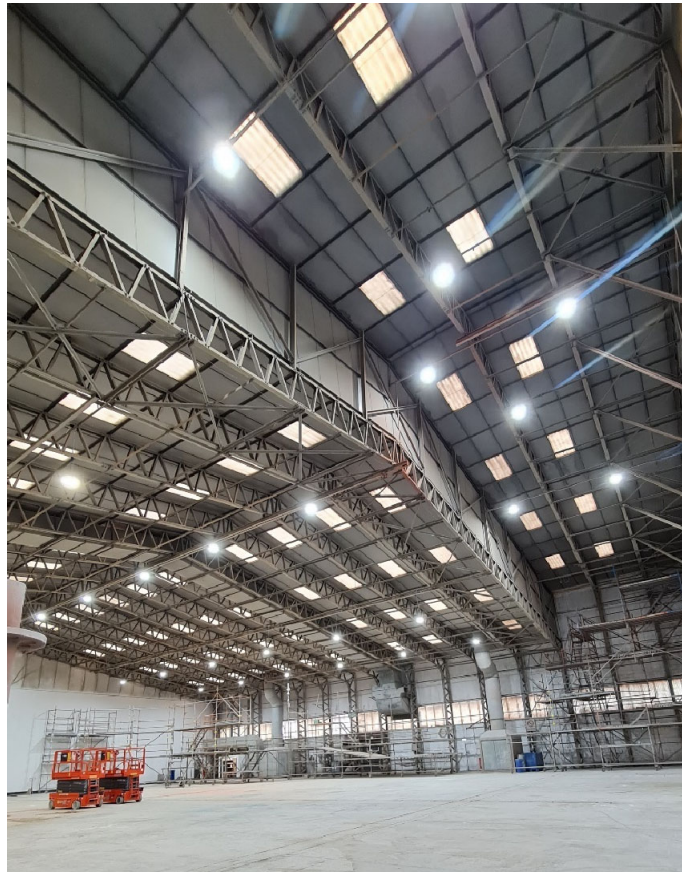
The newly installed LED high-bay lighting. Photograph © Airbourne Colours Ltd
