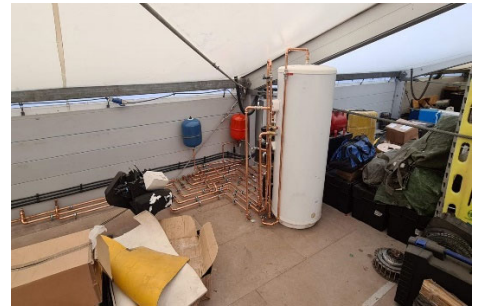
HW cylinder (during installation)
