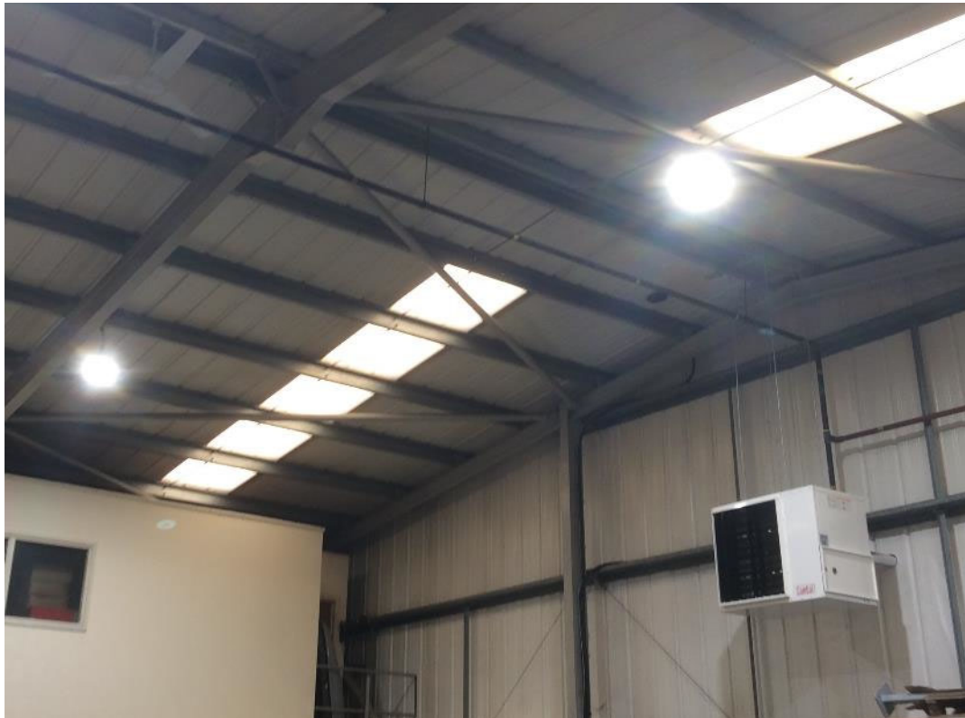
The new LED lighting, gas blower heater and destratification fans installed at Sapcote Engineering Limited
