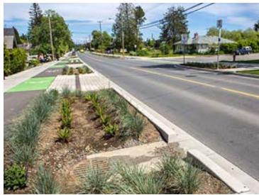
Low-level rainwater garden
