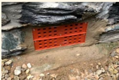
Photo: Automatically closing airbrick, Swithland
