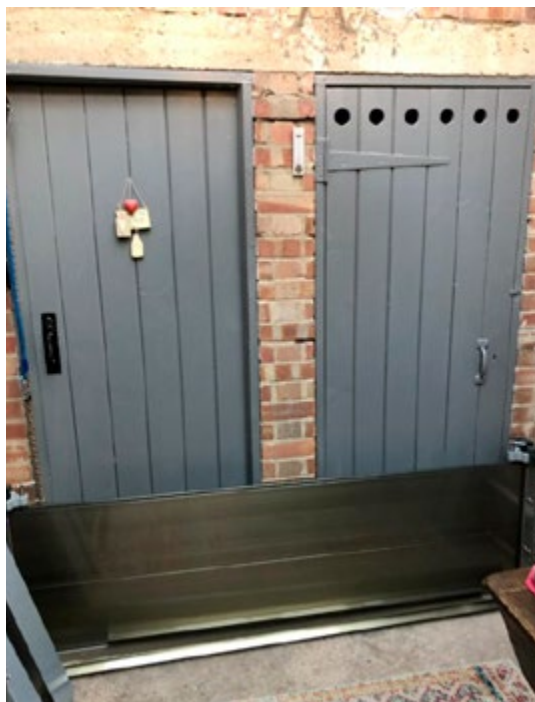
Photo: flood barrier covering two doors, Swithland
