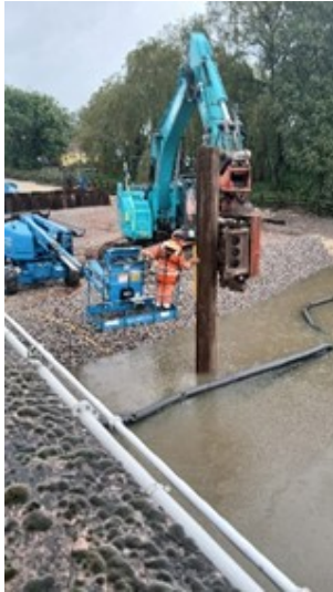
Sheet Piling on the east side of the river to create a cofferdam for the east pier base.
