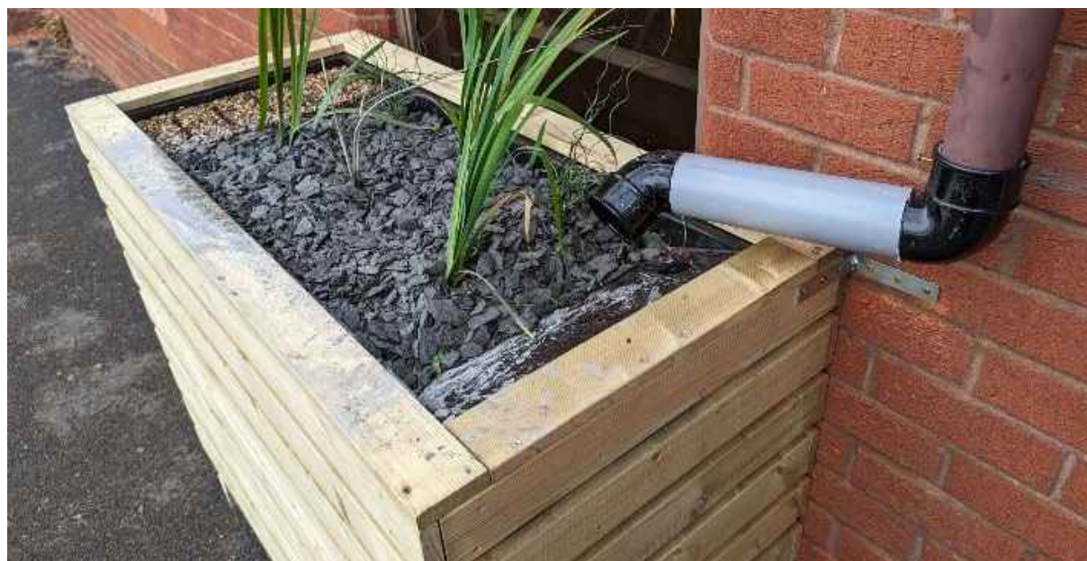
Photo 4.1 – SuDSPod installed at Kibworth Mead Academy (2024).
