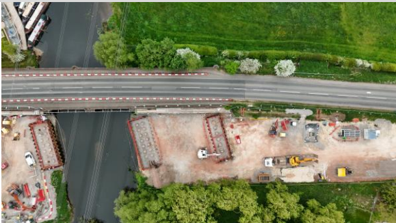
Cofferdams for the two piers and the east abutment. Aerial view of the west pier and cofferdam adjacent to the existing carriageway and Loughborough Boat Club
