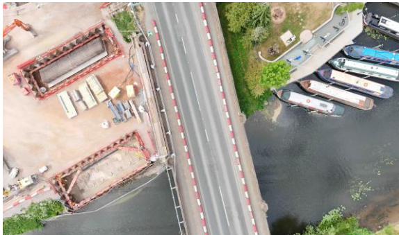
Cofferdams for the two piers and the east abutment. Aerial view of the west pier and cofferdam adjacent to the existing carriageway and Loughborough Boat Club
