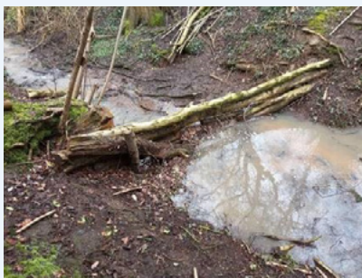
Woody debris fixed into a watercourse to help manage local flood risk
