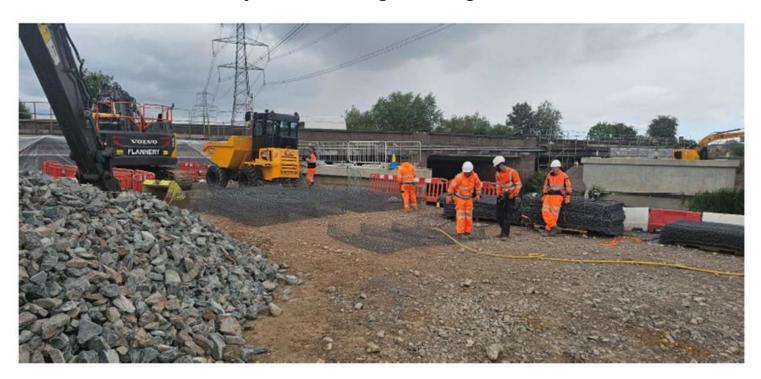
7. East riverbank preparation for revetment mattresses, next to concrete abutment.
