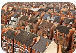
Housing development is supported by the infrastructure
