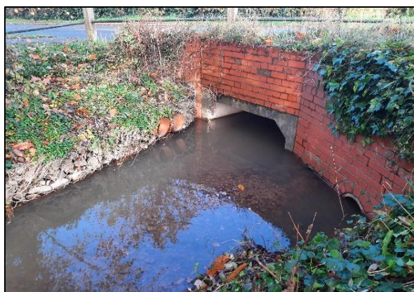
Photograph 6: deposits from upstream in ordinary watercourse 1 downstream of outlet adjacent to 1 Heather Lane
