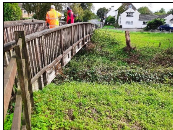
Photograph 12: Illustrating the channel width just downstream of the twin arch bridge
