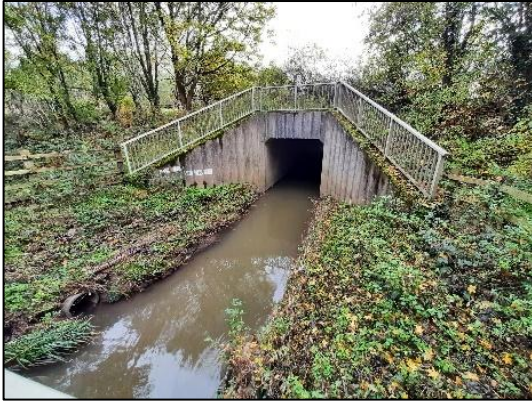
Photograph 1: Upstream of A42 showing bridge inlet and incoming drainage pipe
