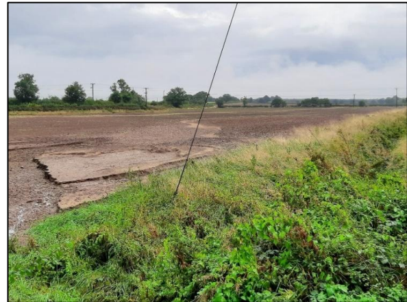
Photograph 5: Taken after the flood event on site visit of 26th September 2023 illustrating scour across land and ploughed fields adjacent to ordinary watercourse 1 upstream of residential dwellings
