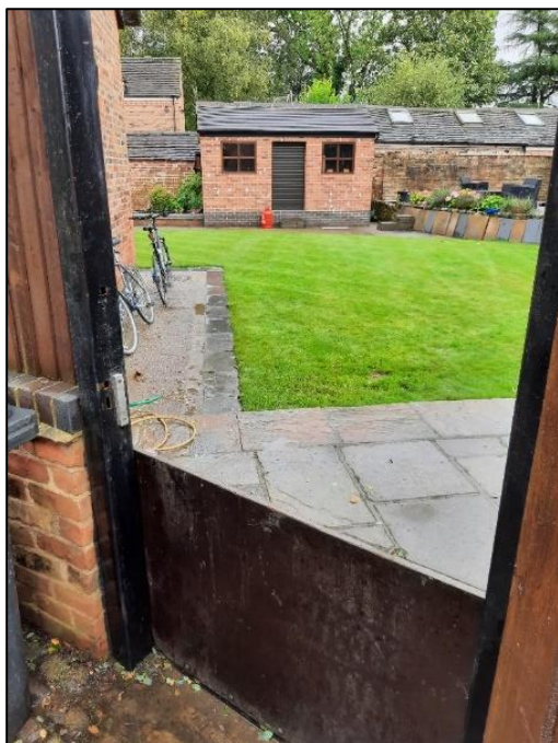
Photograph 13: Makeshift barrier to rear of 53, Mill Street
