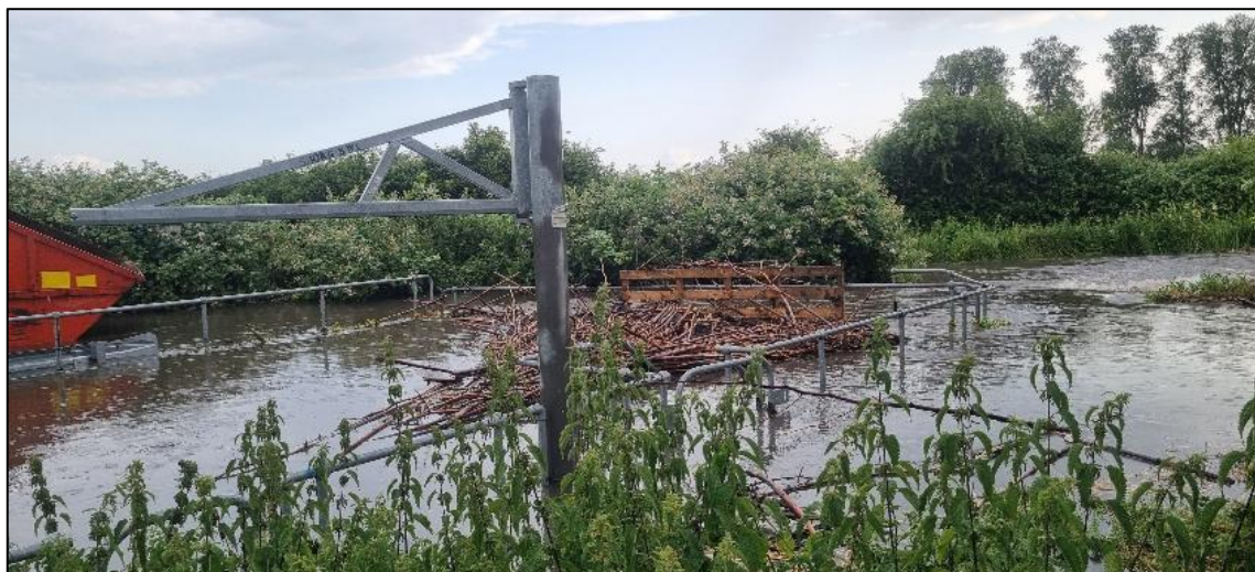
Photograph 24: Blinded screen on storm drain south east of Narrow Boat Close
