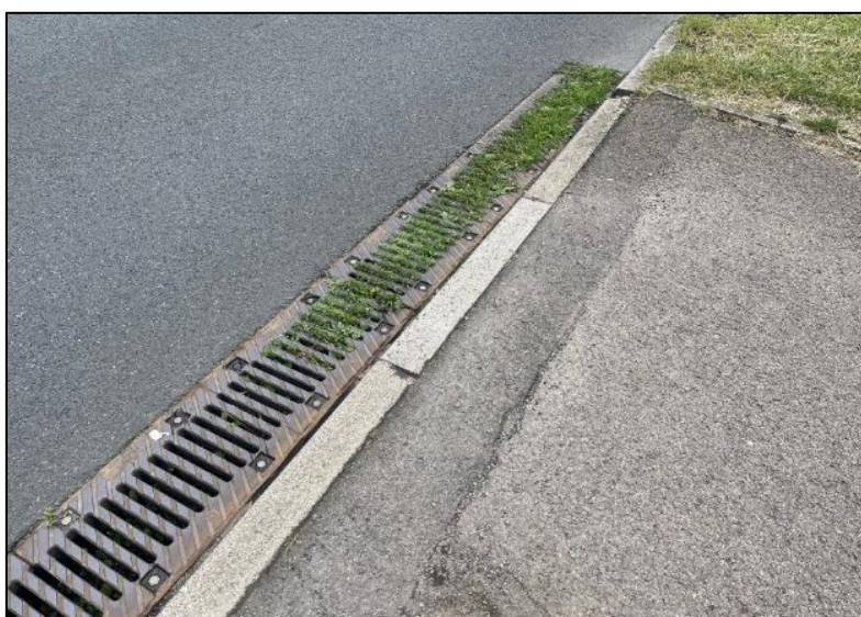
Photograph 13: Partially blocked concrete dished channel drain along Wigston Road
