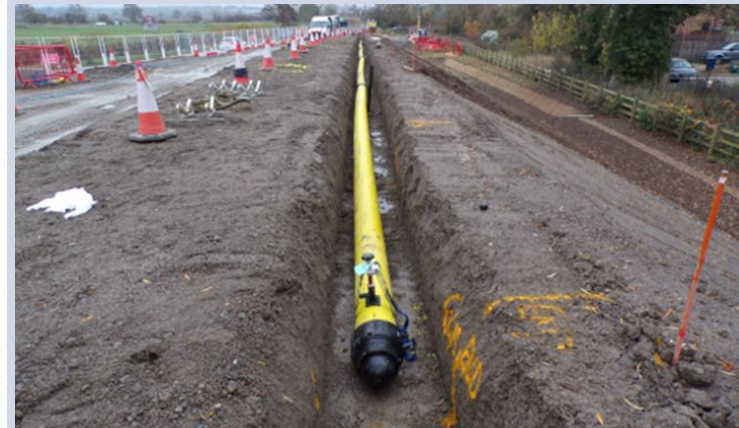
Gas pipe being laid in trench at top of embankment on east side of river. Topsoil has been laid on the embankment slope in the background.
