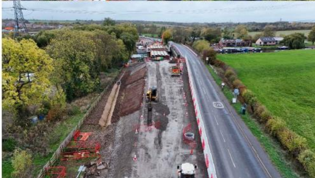
Gas pipe being laid in trench at top of embankment on east side of river. Topsoil has been laid on the embankment slope in the background.
