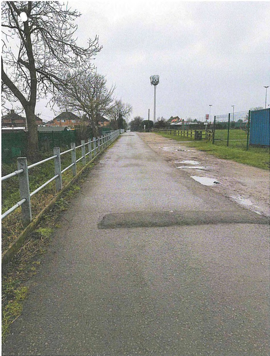
PHOTO TWO MEADOW LANE LOOKING WEST FROM COUNTRY PARK SHOWING SPEED BUMPS INSTALLED BY LCC
