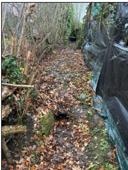
Photograph 4-3: High-level ditch / culvert – December 2025
