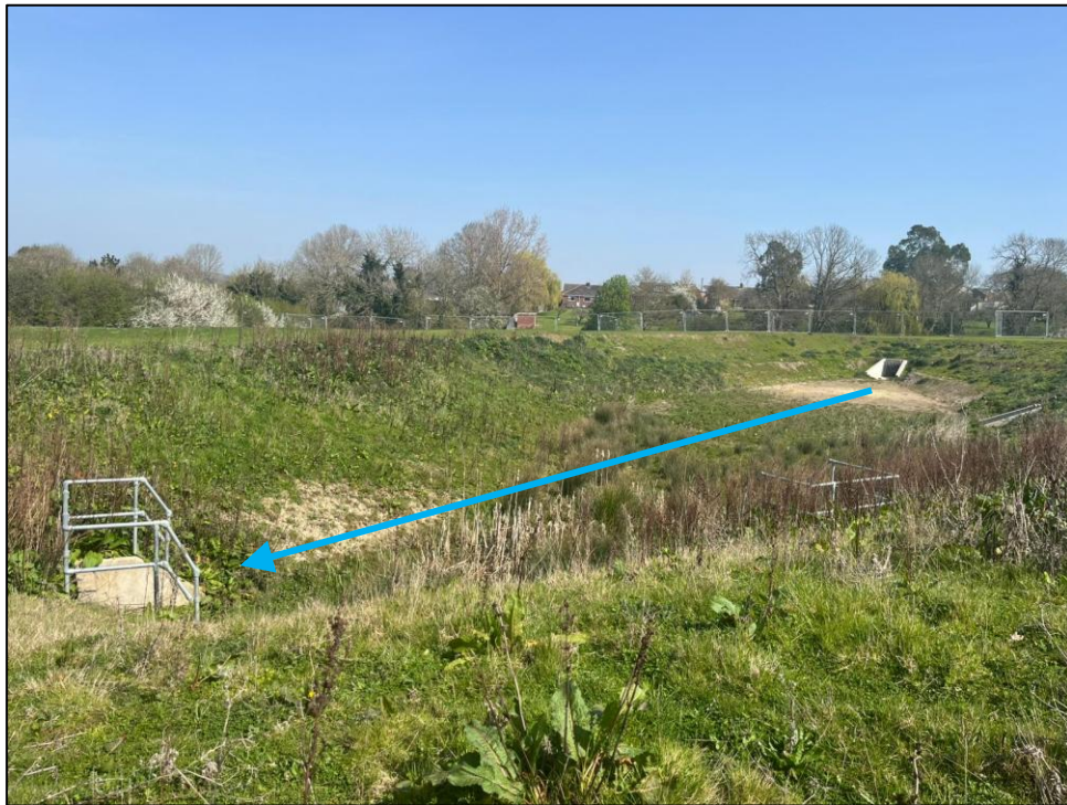
Photograph 6-2: Rotherby Manor Eastern Balancing Pond and Out-fall Headwall into Ordinary Watercourse 1
