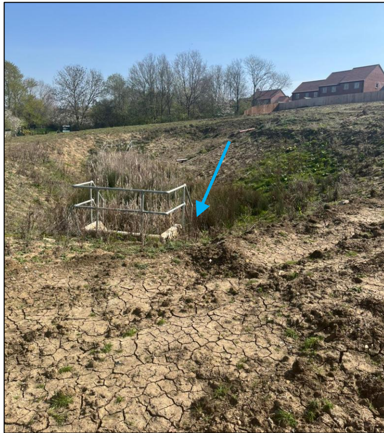
Photograph 6-3: Rotherby Manor Western Balancing Pond and Outfall Headwall into Ordinary Watercourse 3
