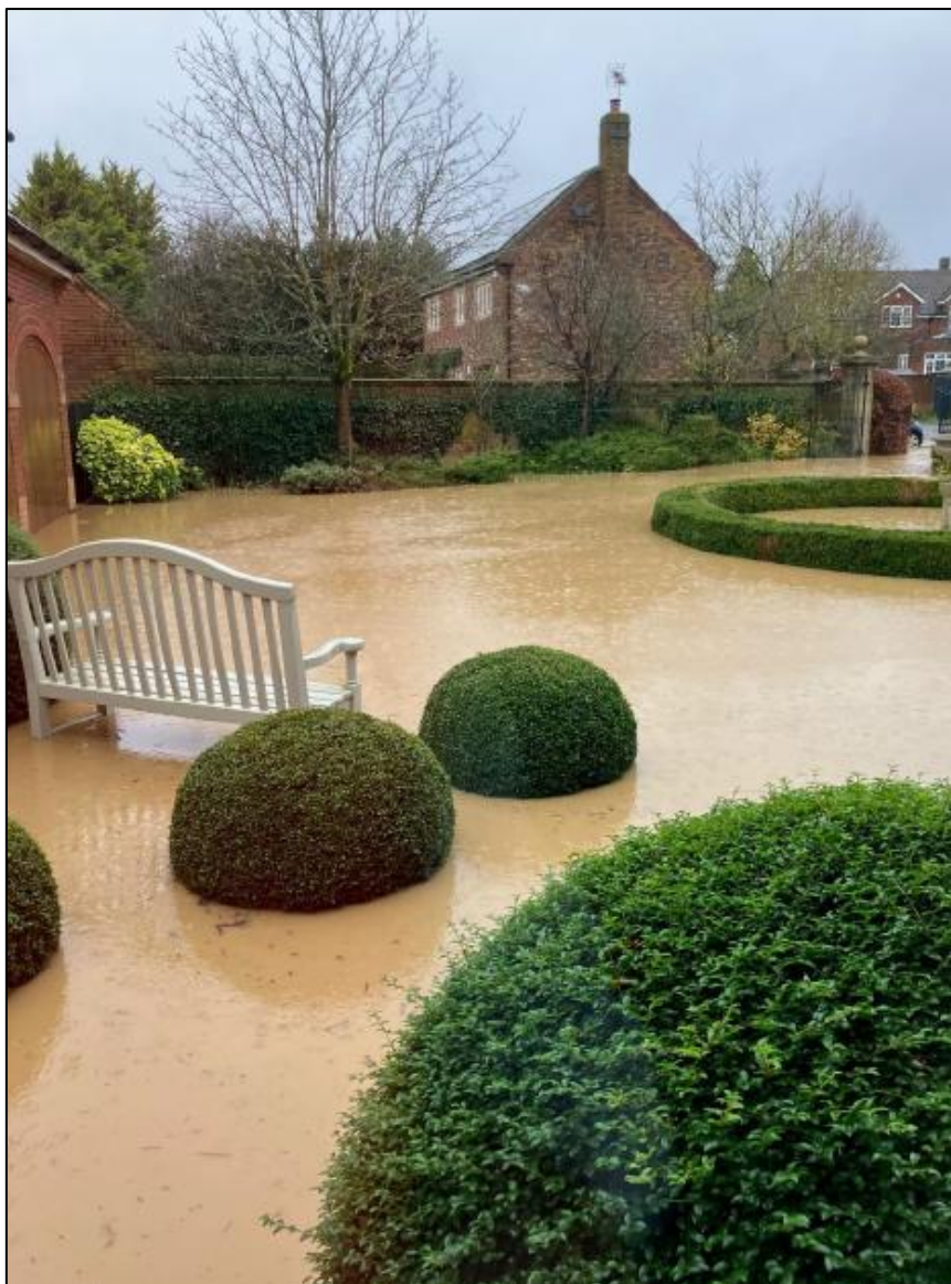
Photograph 7-11: Garden flooding along Bluebell Lane
