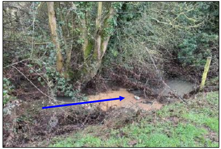
Photograph 7-9: Vegetation debris within Glooston Arm channel 3
