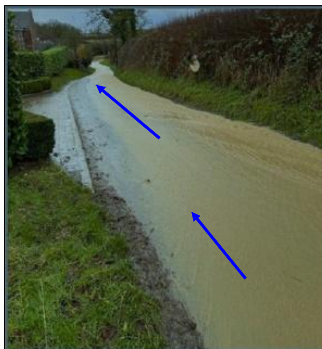
Photograph 7-3: Surface water flowing down Goadby Road towards Glooston village centre
