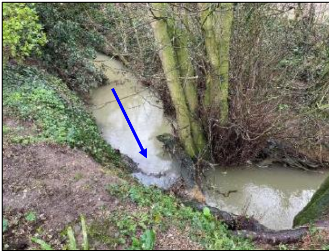
Photograph 7-8: Vegetation debris within Glooston Arm channel 3
