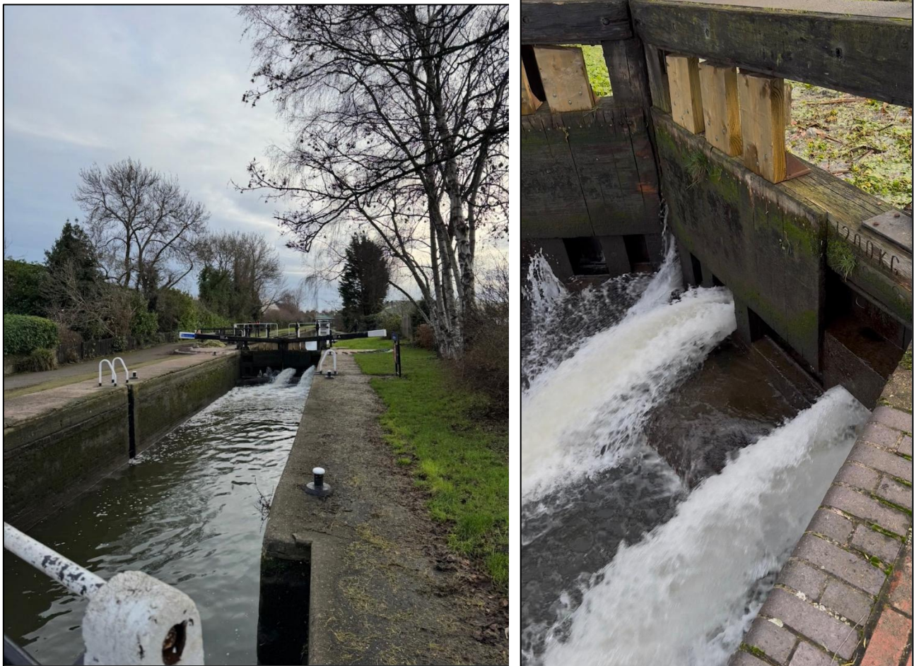
Photograph 8-10: Loughborough Lock 53 drawdown procedure in progress by Canal and River Trust
