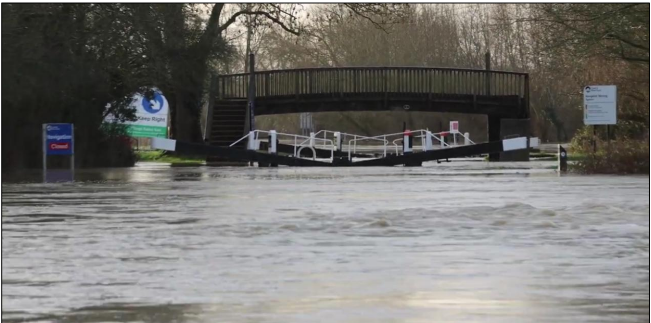
Photograph 8-3: Inundation of the Grand Union Canal at Pillings Lock on the Morning of Wednesday 3rd January 2024
