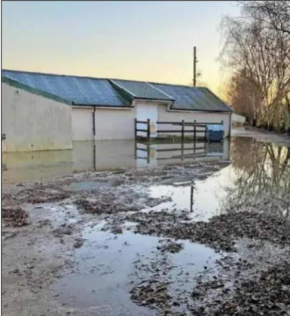
Photograph 8-2: Aftermath of flooding at Carillon Sports Club 13
