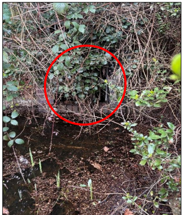
Trash Screen on Culvert Inlet Credit: Simon Austin
