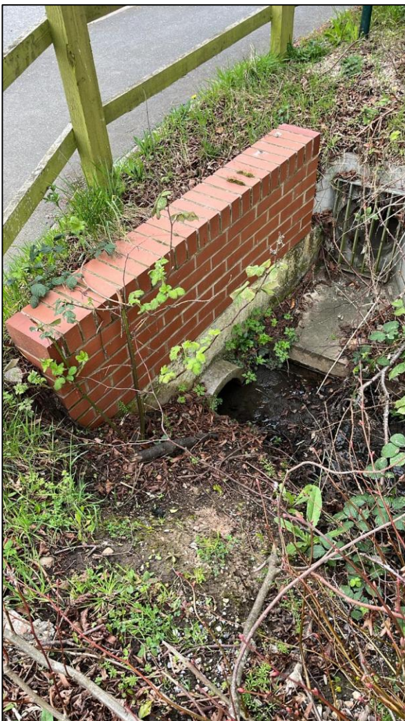
Photograph 17-1: Culverted Ordinary Watercourse 2 Outfall on northern side of Butler Close (Location B)
