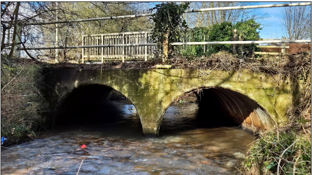
Photograph 11-1: The Dog and Gun Lane Twin Arch Bridge
