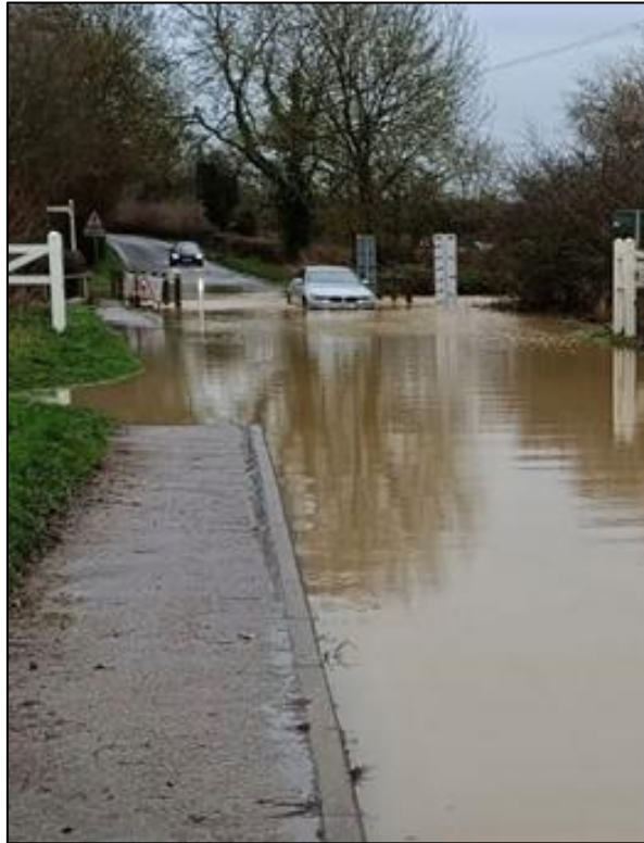
Photograph 20-7: Flooding at Wymondham Drift – depth shown on flood gauges
