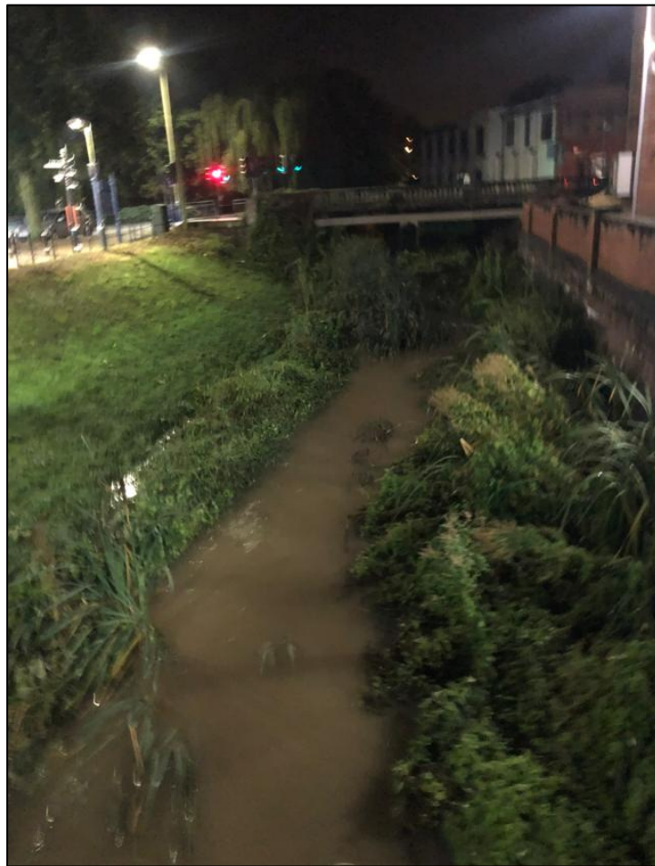
Photograph 3-8: River Welland viewed upstream towards Northampton Road bridge at 20:30 hours BST
