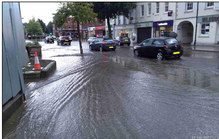
Photograph 3-5: Flooding along High Street at 17:54 hours BST
