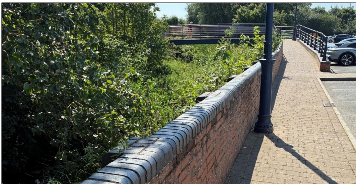
Photograph 3-1: Raised Flood Defence in The Commons car park, Market Harborough Town Centre (7 th July 2026)
