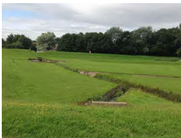
Photograph 3-4: Eastern Catchment 'Winter' Basin
