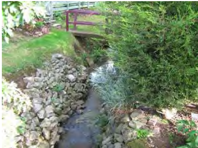
Photograph 4-3: View downstream towards constriction adjacent to flooding location at Shakespeare Close
