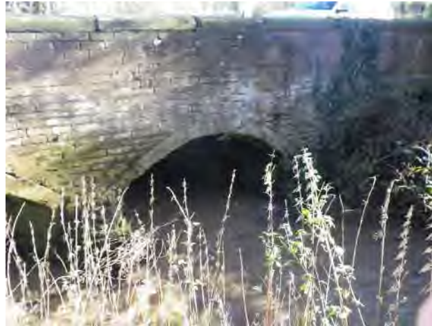
Photograph 4-8: Brick Arch Culvert
