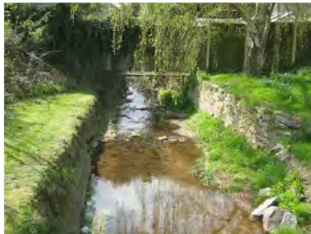
Photograph 4-2: View looking upstream from culvert
