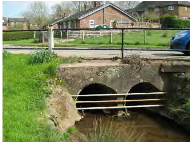
Photograph 4-1: Upstream view of the Bowley culverts
