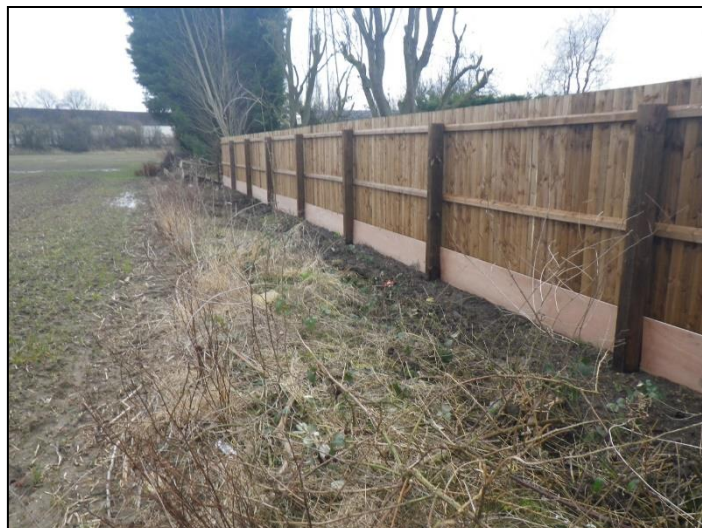
Figure 7: The ditch to the rear of properties on Watling Street. A small depression was still present however capacity has been severely reduced.
