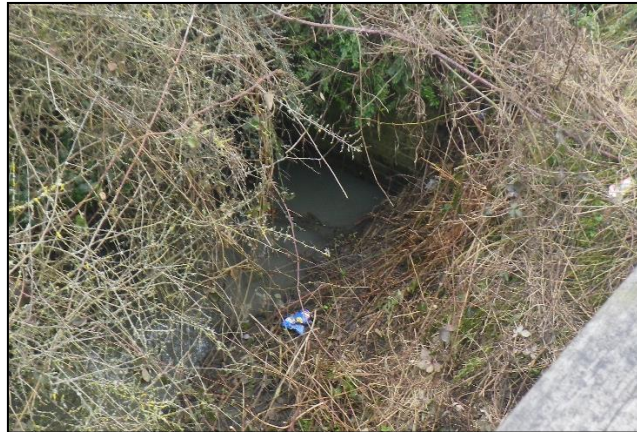
Figure 6: The highway system outfall the day following the flood event. The outfall is still submerged and poorly positioned to discharge effectively
