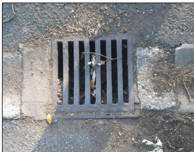
Figure 5: The pavement gully outside the affected properties (taken after the event illustrating siltation)
