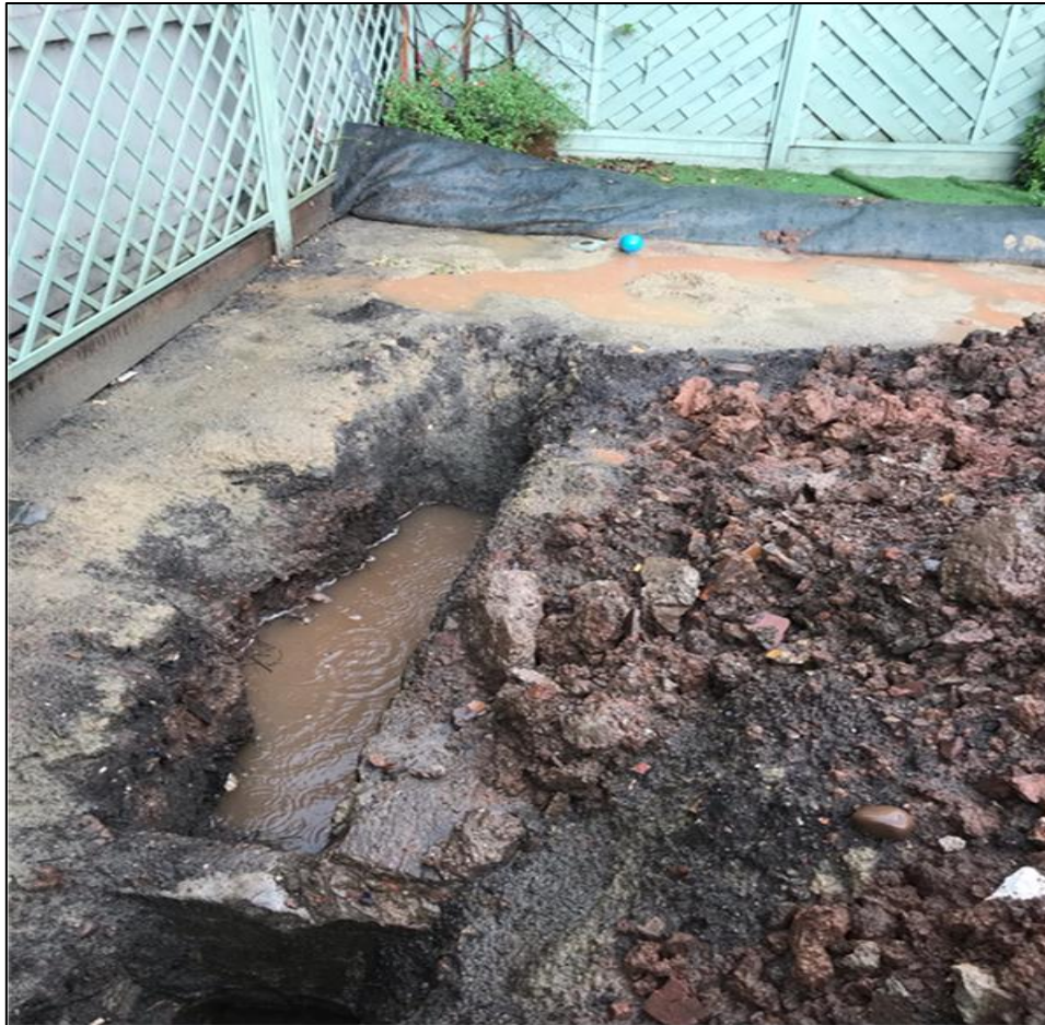
Picture 5: Water collecting in Land Drain A (No. 20) due to the drain being severed to rear of the property in Sherwood Court
