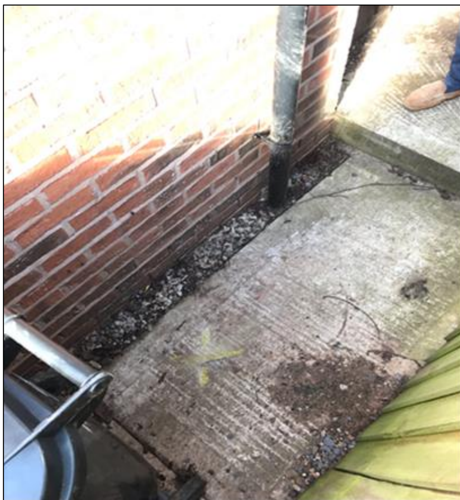
Picture 7: Yellow 'X' denotes location where Land Drain B running from No. 16 West End is severed at property to the rear in Sherwood Court
