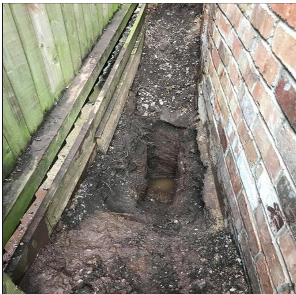
Picture 6: Water collecting in Land Drain B due to drain being severed where it leaves the property (No.16) and meets the property to the rear on Sherwood Court
