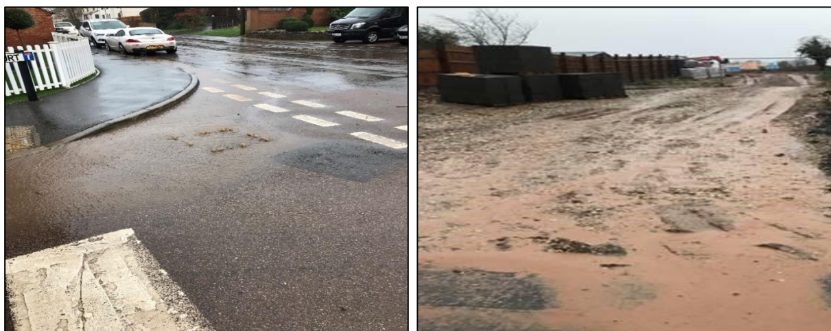
Pictures 1 & 2: Showing water surcharging from the inspection chamber in Sherwood Court (from a later flood event) and surface water flowing onto West End from the live construction site on 14 th November 2019
