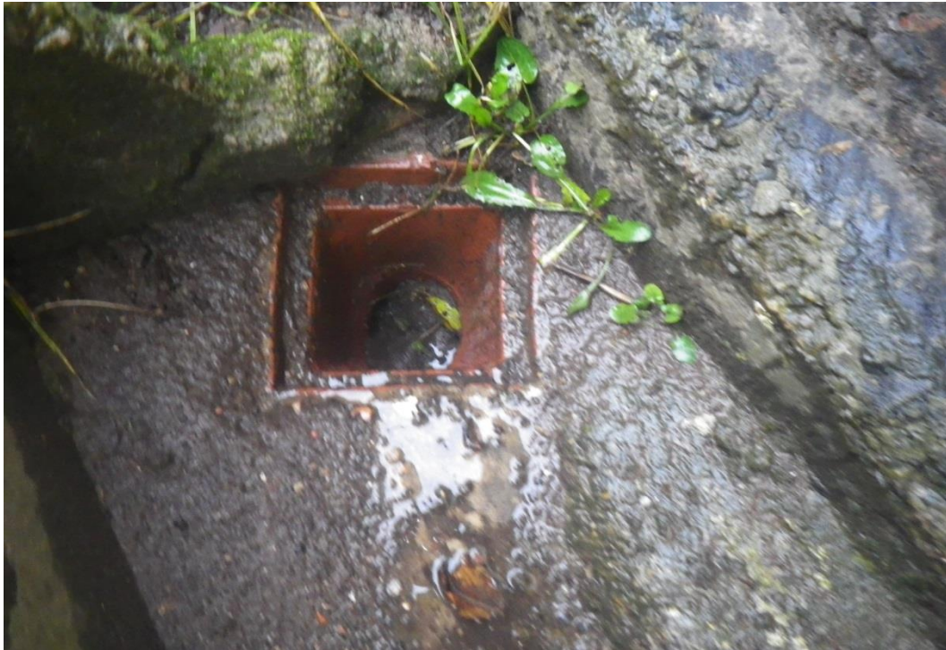
Photograph 2: Blocked connecting pipe at the end of the trench
