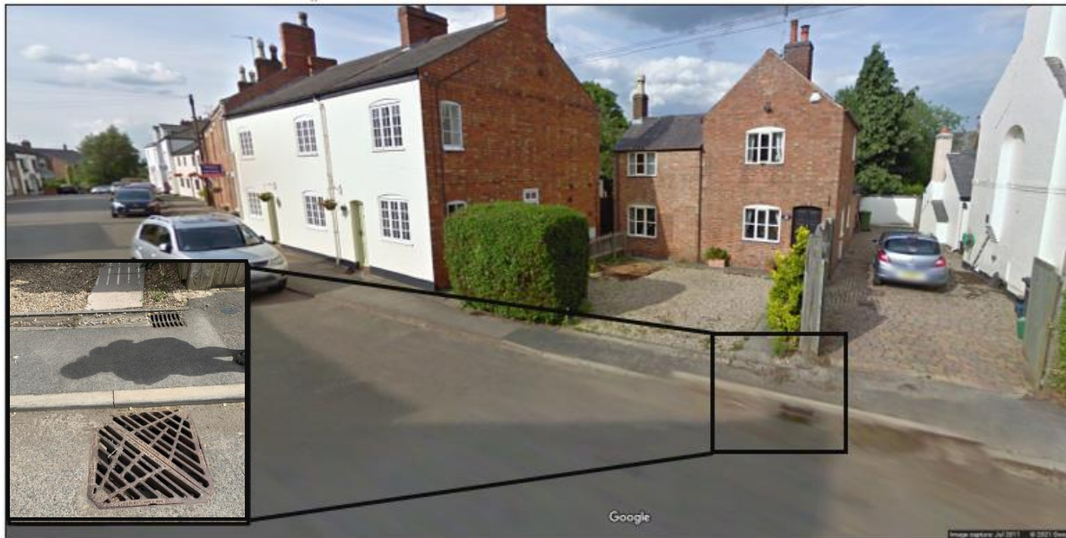
Photo 6: Small concrete concave channel which runs along the front of the impacted residential properties (main photo taken from Google Maps in July 2011 and small photo taken in May 2021).
