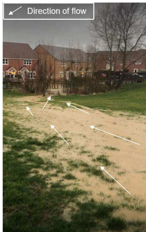
Photo 2: Surface water flow path from the development site easterly boundary towards homes on Buckthorn Way (downhill view)
